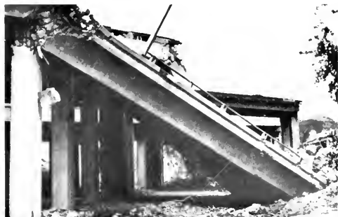
Photo 4. Southern portion of the San Fernando Road overhead [2].
